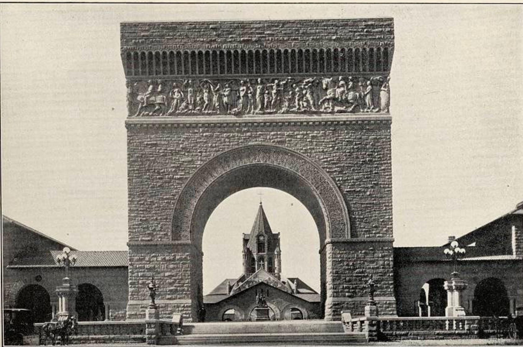
ILL. No. 65. MEMORIAL ARCH, WITH CHURCH IN BACKGROUND, STANFORD UNIVERSITY, SHOWING TYPES OF CARVED WORK WITH THE SANDSTONE.
