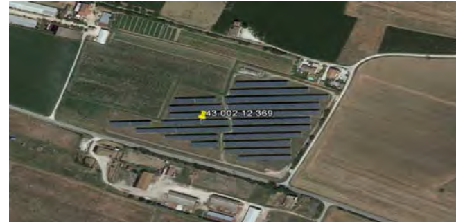
Italy; 1.935 MW Fixed Array
