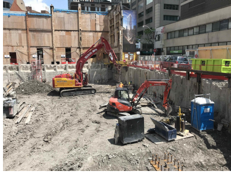
Figure 10: CLIP Model Predictions: MINI_EXCAVATOR, EXCAVATOR, DRILLRIG, TIEBACK_RIG, DOZER; Visual Encoder Decoder generation: an image of excavator tieback rig power generator.
