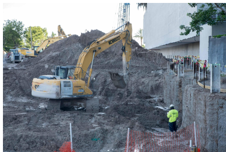
Figure 4: An image of excavator and skid steer
