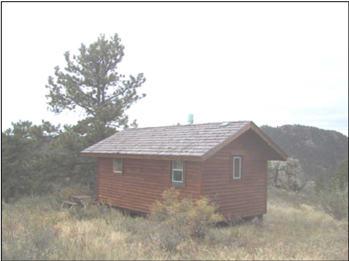
Fig. 2. Cabin near Virginia Dale, CO, looking approximately southwest (north and east walls of cabin). Photo taken September 2001.
