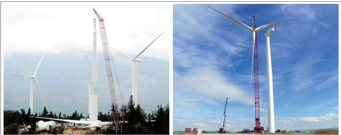
Figure A3: Modular tower sections and ground-level rotor assembly
