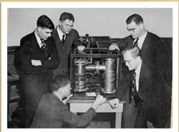
Russell Varian (1899-1959), left, and Sigurd Varian (1901-1961) appear in this 1951 photograph with a high-powered klystron. In the palm of his hand, Russell Varian holds a smaller type of klystron used for radar, aircraft instrument landing and microwave communications. (co-founders of Varian Associates in 1948)
