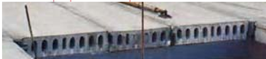
Floor Slab Span - 6.7m 0.2m Thick Hollow Core
