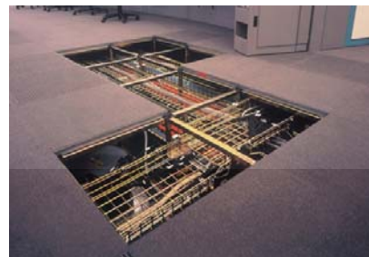
Raised Flooring for Third Floor
