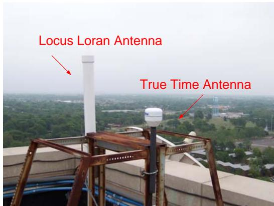
Figure 8: Locus Loran antenna and True Time GPS antenna in Norman, OK
