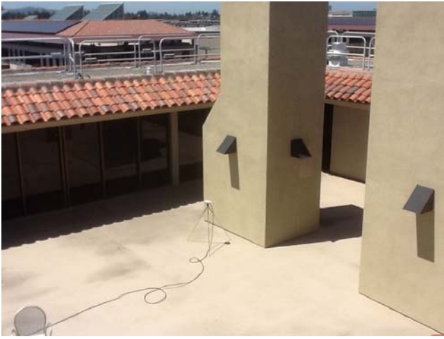
Figure 11. Durand Building Roof Courtyard (4 th Floor)
