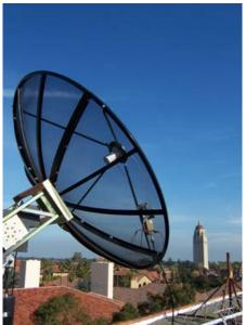
Figure 1. The SGMS 1.8 m dish antenna
