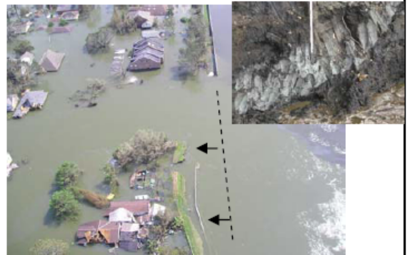
Displacement of wall and part of levee
