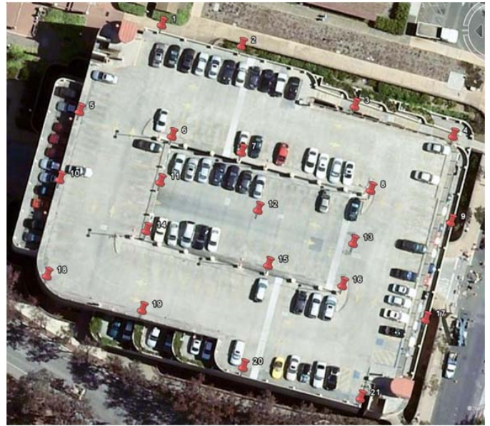
Fig. 7. Roof of Mitchell Building in Stanford University
