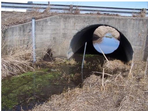
Figure 39: Wagner Gage Site, Showing Stilling Well (March 2006)
