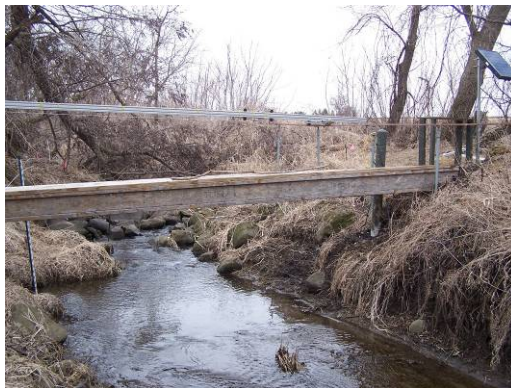
Figure 42: Kippley Gage Site, Showing Stilling Well (March 2006)
