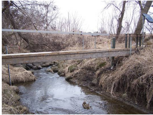
Figure 34: Typical S1 Cross Section (at Kippley Gage, March 2006)
