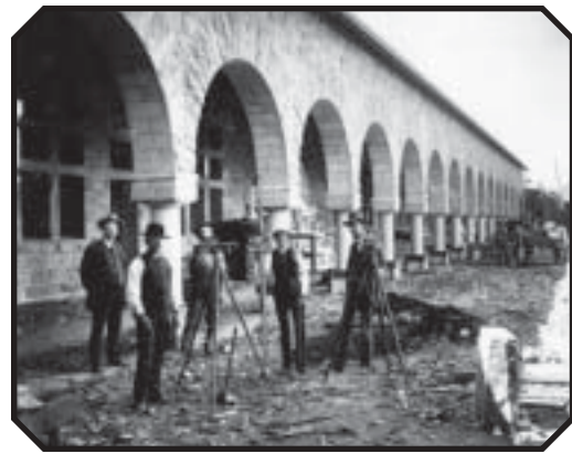
Construction of the Quad
