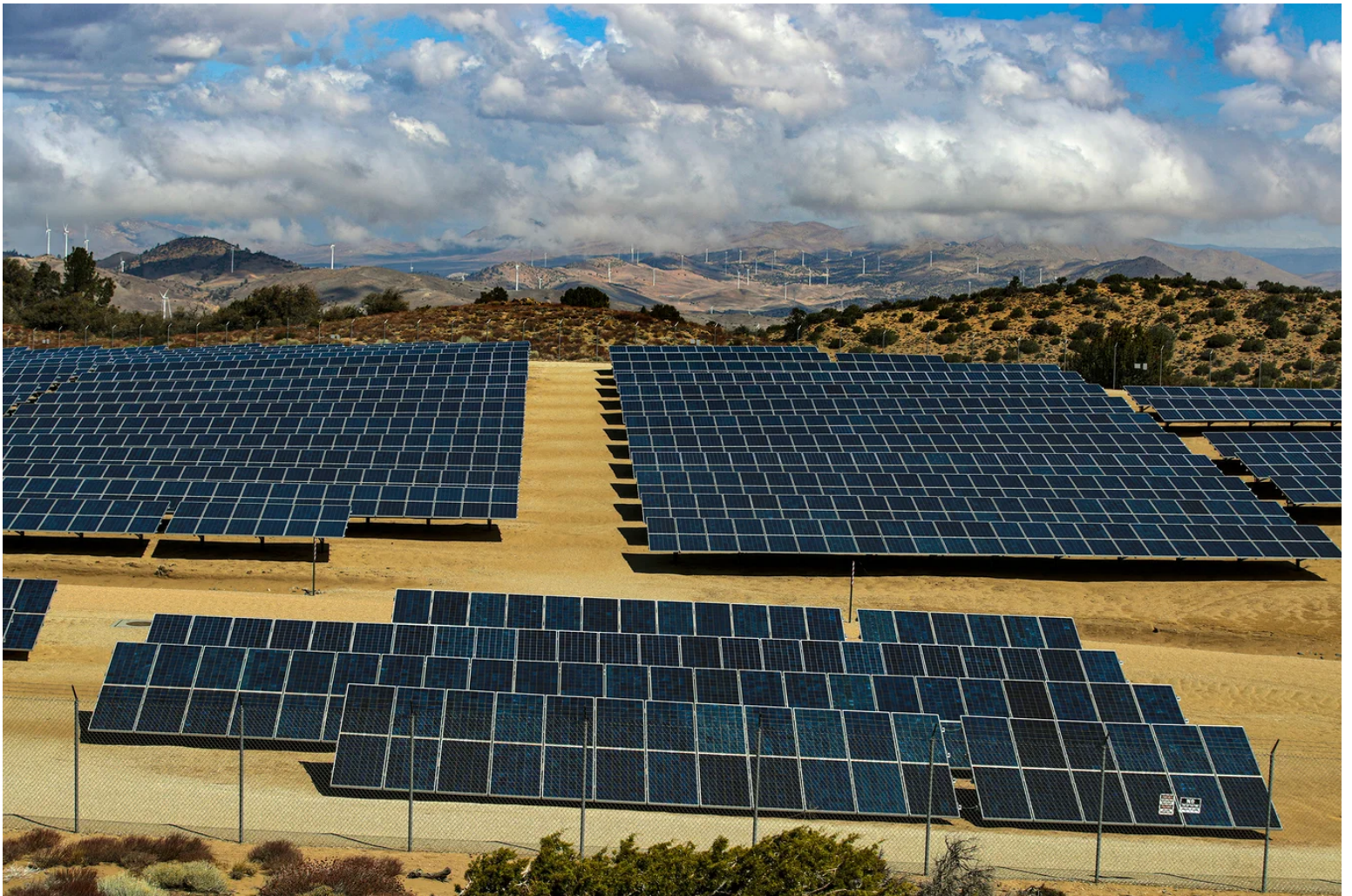
LADWPs Pine Tree Wind Farm and Solar Power Plant in the Tehachapi Mountains of California. Irfan Khan/Los Angeles Times via Getty Images
