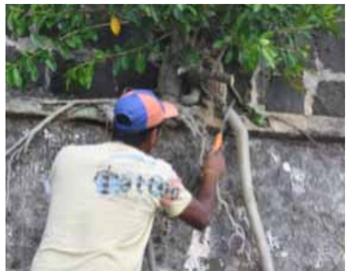
Emergency measures undertaken to remove vegetation in the barracks © AGTF
