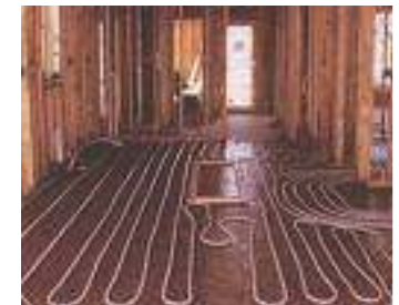
UFHH (Under floor hydronic heating)
