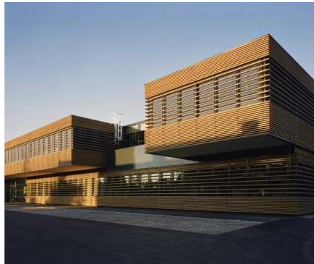
Poppe Prehal – Engineering School Mistelbach
