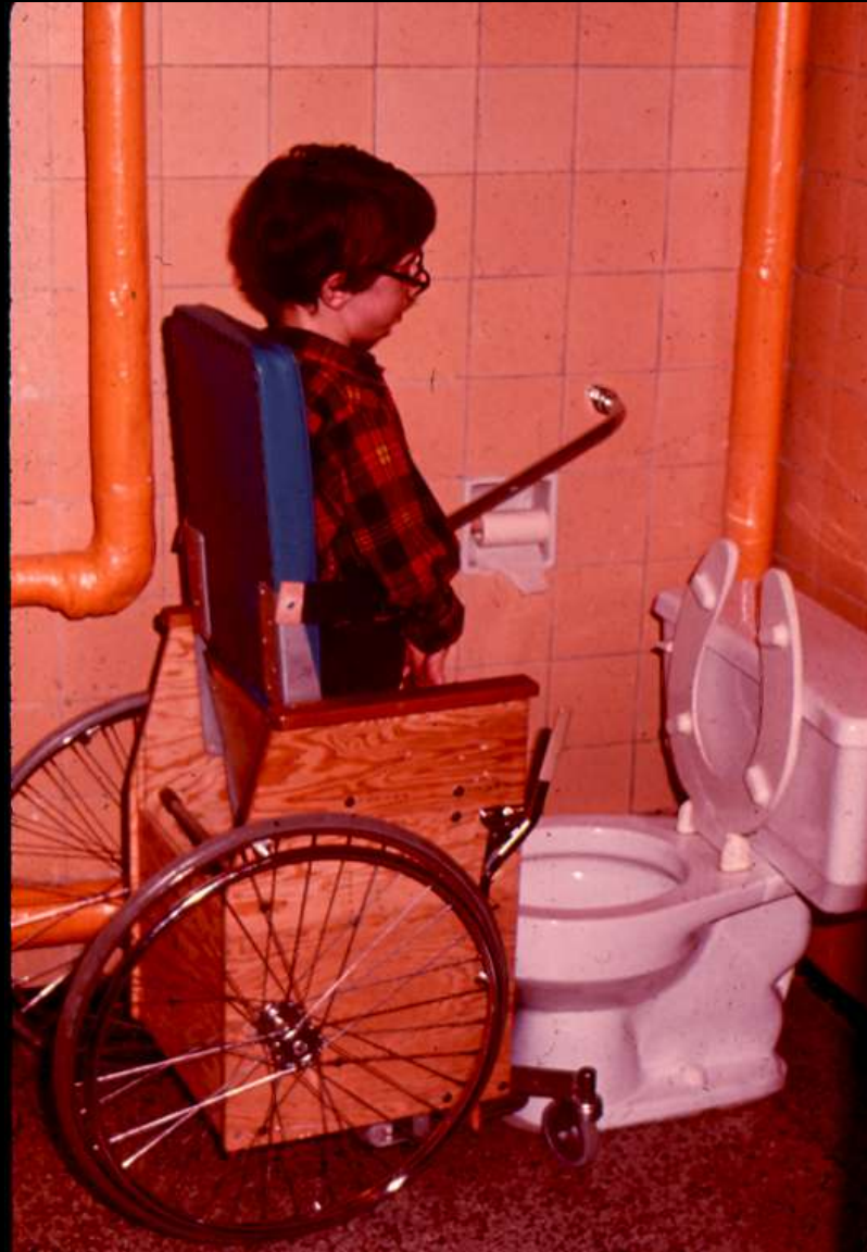
Stand Up Wheelchair Prototype – Early 1970s
