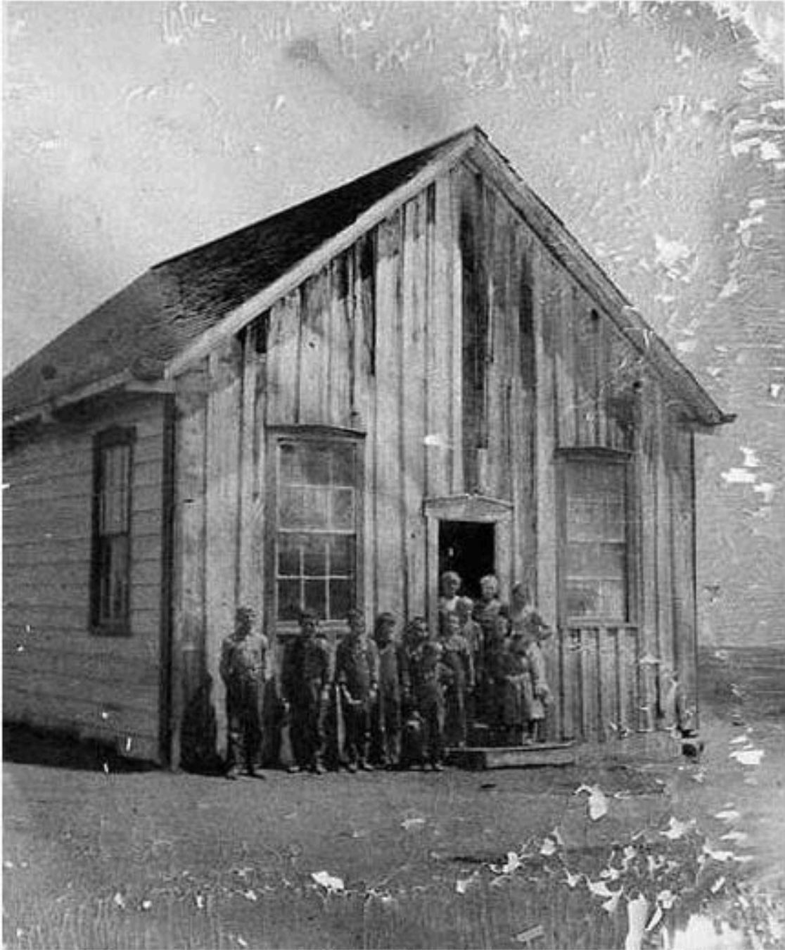
Warm Springs School, the first schoolhouse at Paraiso Springs, built in the 1880's. From "Revised Evaluation of Historical Resources at The Paraiso Springs at 34358 Paraiso Springs Road in The County of Monterey"
