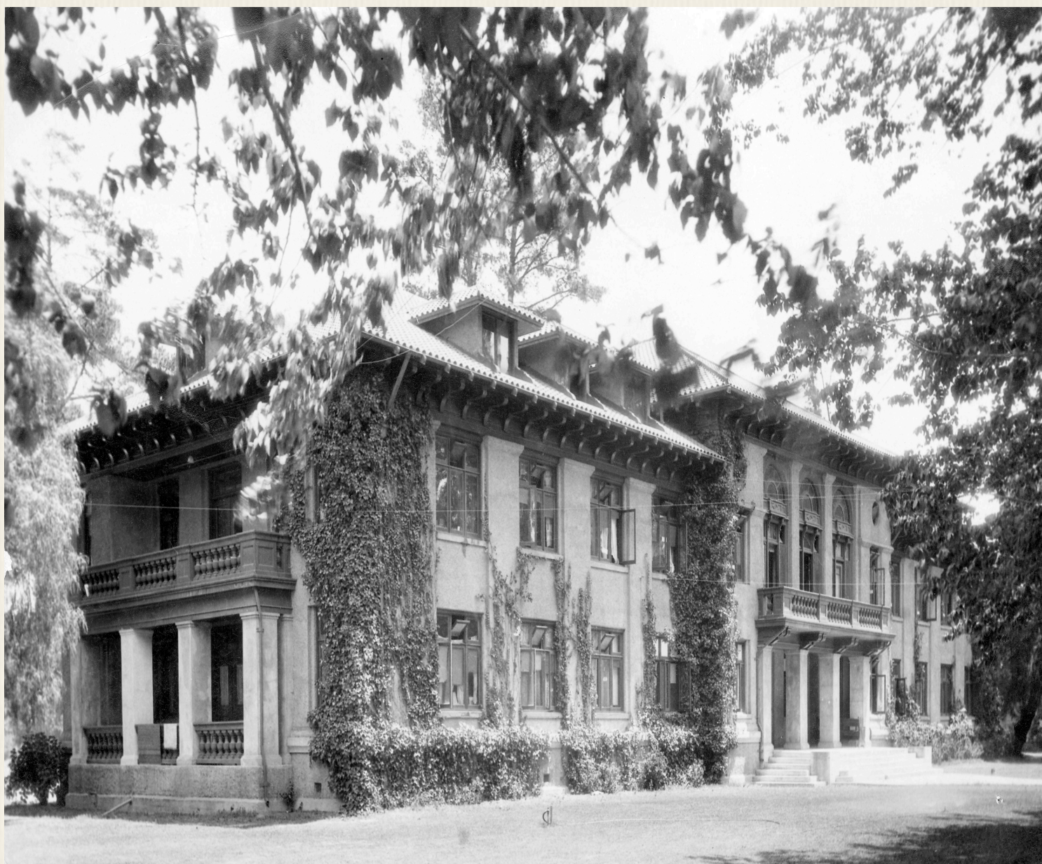
University of the Pacific in San Jose. Photographer: John C. Gordan Photograph courtesy of the San Jose State University Library Special Collections and Archives.
