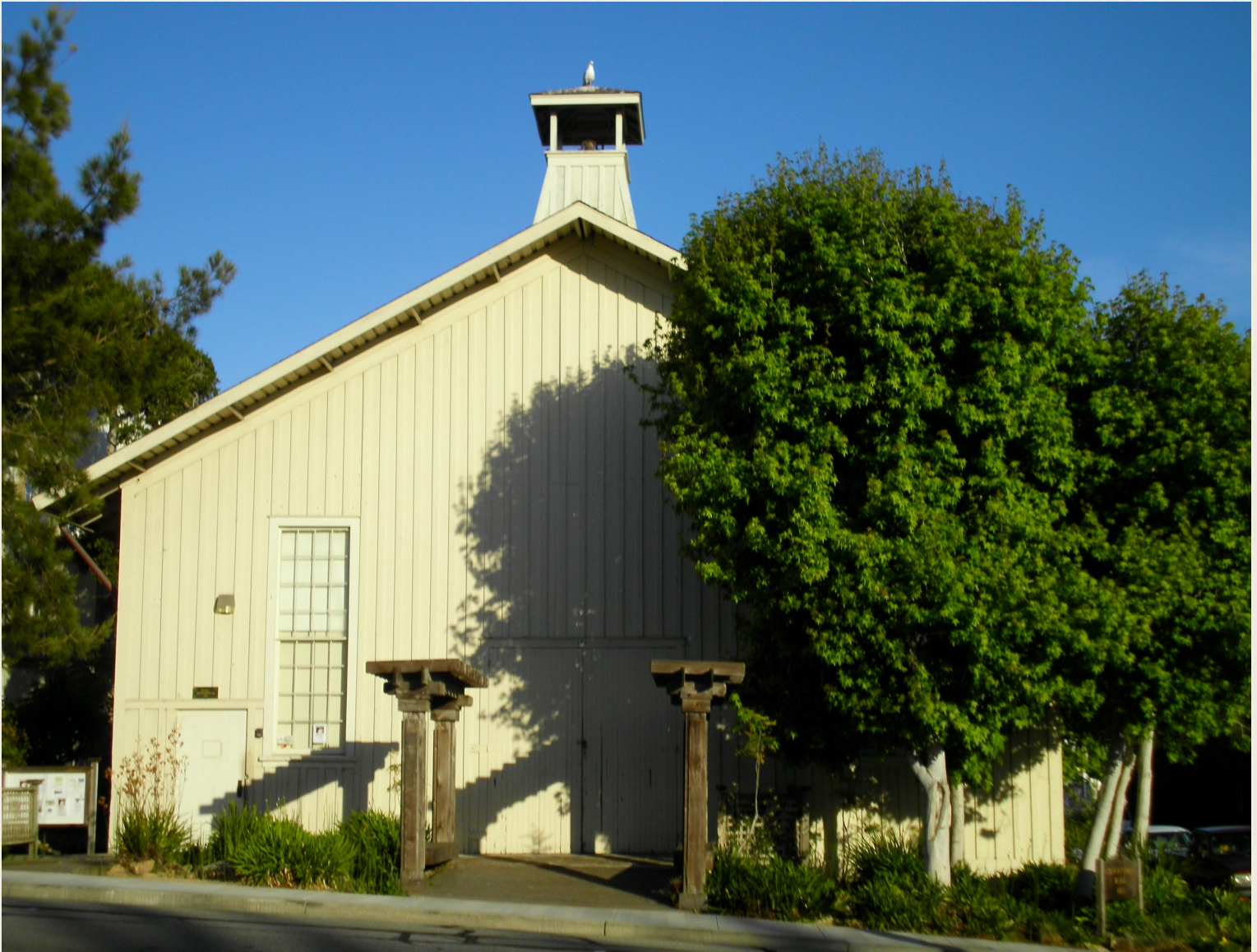
Hall in the Grove (or Chautauqua Hall) in Pacific Grove, California. c2014.
