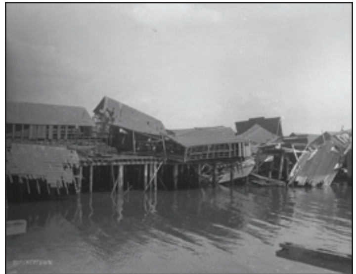
Figure 4 | The stilted structures of Butchertown after massive damage from the 1906 earthquake. The slaughterhouses were designed so that offal would fall into the tide below. 23
