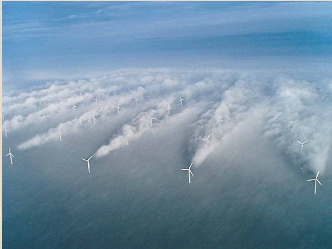
Image above: The above photograph shows the turbulence field behind the Horns Rev offshore wind turbines. Horns Rev is located in the North Sea, 14 kilometers west of Denmark. Photographer Christian Steiness. From ( http://wattsupwiththat.com/2011/04/28/the-wind-turbine-albedo-effect/ ).
