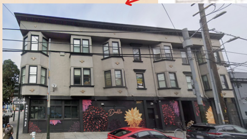
Preserving this building
