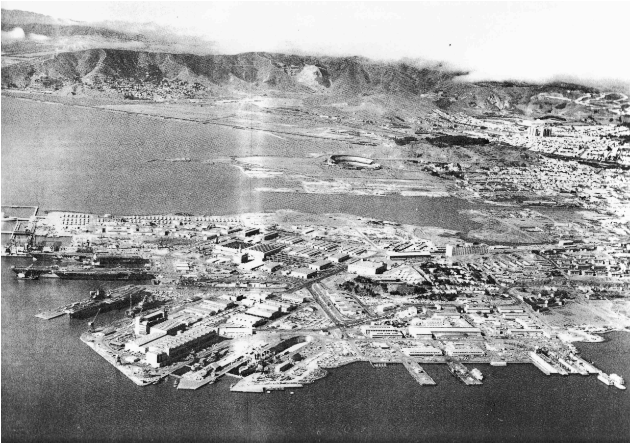
Figure 3: Arial View of the Hunters Point Shipyard, 1966.
